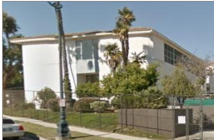
Photograph 3 – Southern and Eastern Elevation (looking North-West) Building D; taken April 2013 (via GoogleMaps.com)
