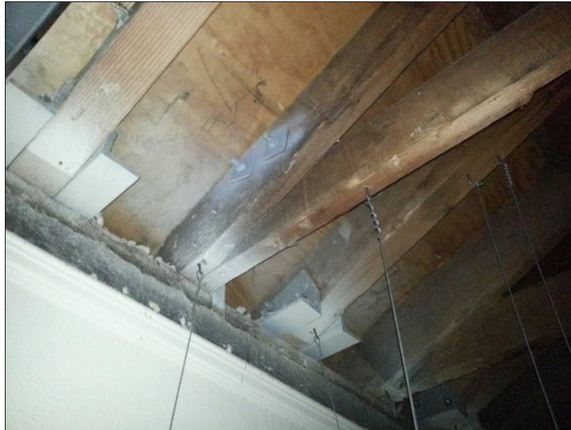
Picture 5 – Roof to Top of Wall Condition – Building B (showing angle and ply'd retrofit)
