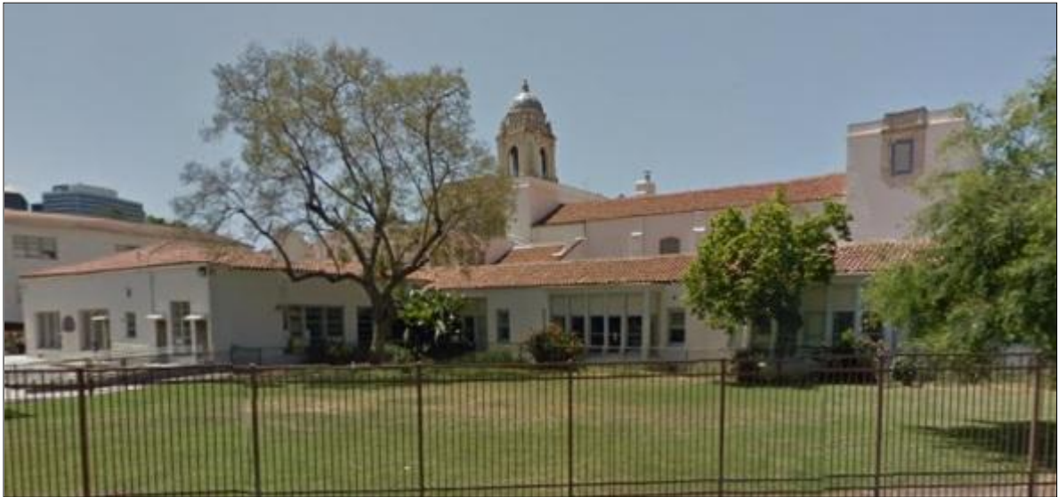
Photograph 2 – Partial Eastern Elevation (looking South-West) Bldg B (low, foreground) and Bldg A (high, background) Taken April 2013 (via GoogleMaps.com)
