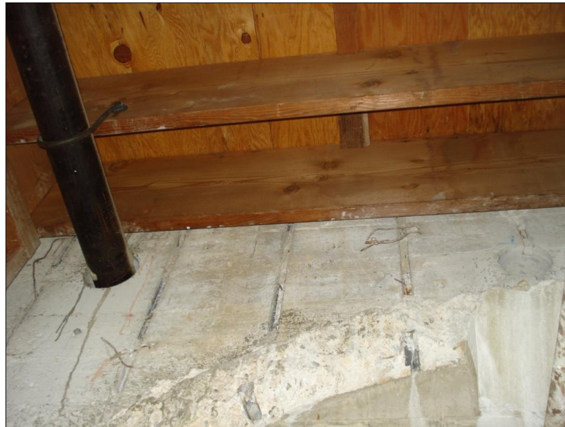
Picture 4 – Building C (conc. wall) to Building D (wood framing) Condition at in Hallway Ceiling Plenum – 1 st Floor (showing seismic separation)
