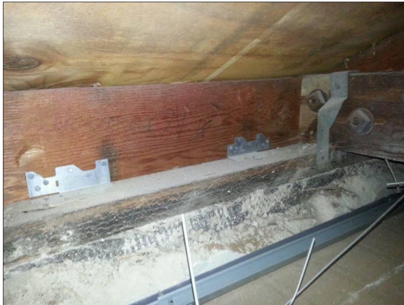
Picture 1 – Top of Wall to Roof Condition in Classroom Ceiling Plenum – Building B (showing Simpson A35 retrofit, ply'd shtg, lack of OOP anch's)
