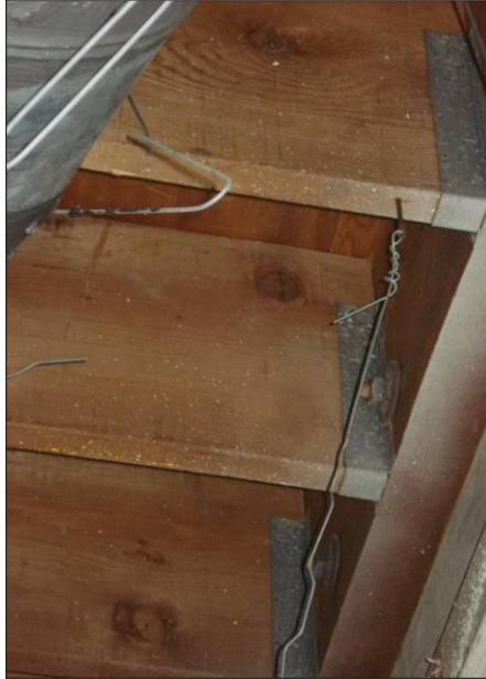
Picture 3 – Wall to Floor Condition in Classroom Ceiling Plenum – Building C (showing lack of OOP anch' s)
