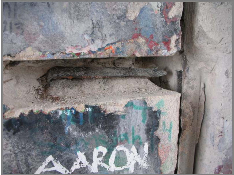
Photo 7 Metal anchor found in mortar joint of cast stone, separated from metal channel embed
