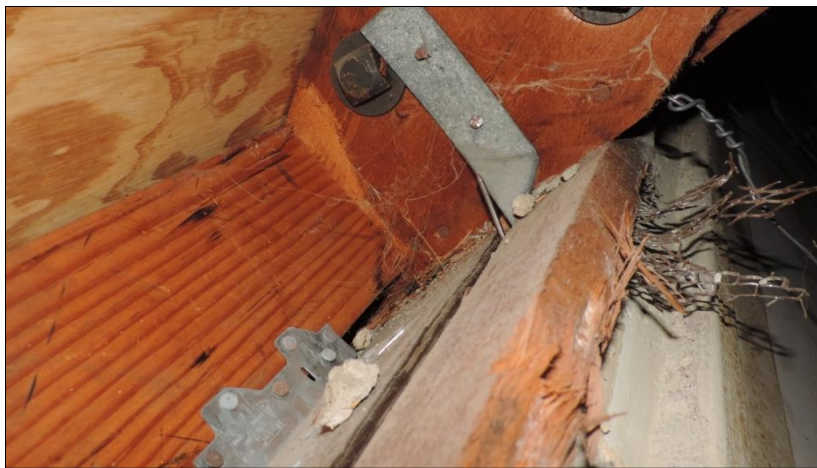
Picture 2 – Top of Wall to Roof Condition in Classroom Ceiling Plenum – Building B (showing Simpson A35 retrofit, ply'd shtg, lack of OOP anch's)
