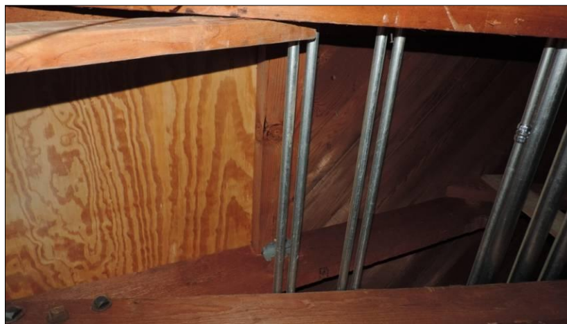
Picture 6 – Roof Plywood Sheathing to Diagonal Sheathing Condition – Building B (showing angle, ply'd, blocking retrofit)
